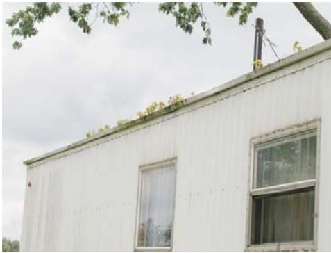
Fig 4. Maple seedlings are a good indication of standing water on this flat roof.
