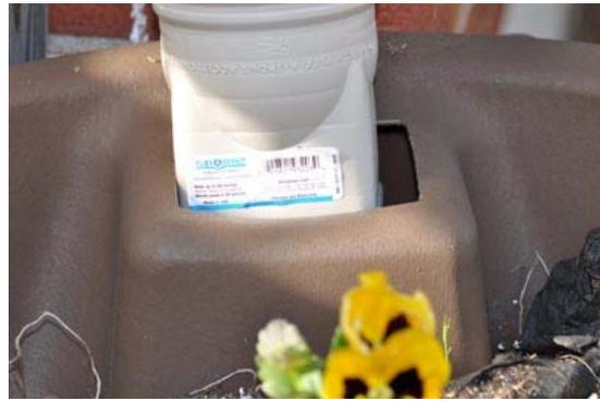
Fig 5. Gap around downspout entry to rain barrel gives mosquitoes access to water.
